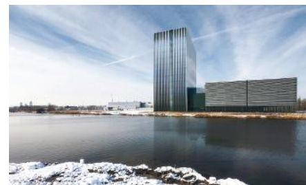
DATACENTER EQUINIX IN AMSTERDAM
