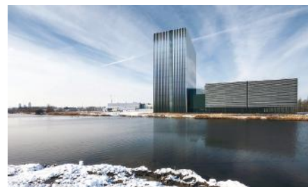
DATACENTER EQUINIX IN AMSTERDAM
